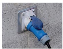
Just a CEE socket must be available: CEE 16A for single-phase devices (blue camping socket) or CEE 32A for three-phase devices (red). No more expensive installation is needed.
